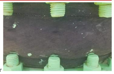
clarifiers. The expansion joints were delaminating and showing fabric reinforcement around the bellows. They reached out to a Holz Distributor to assist them in finding a long term solution that would eliminate these problems in the future.
