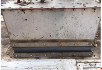
solution using their 945 style designed to allow much more significant movement than the joint that had torn open. The 945 design is a fully molded expansion joint with a bellows in the body of the joint that allows maximum movement without stressing the system. Our Engineered solution helped the plant to get running again and will ensure safe and leak-free operation.
