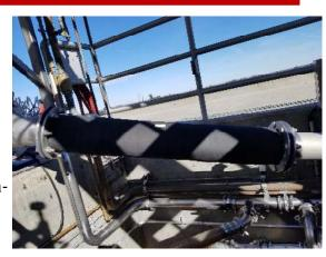
tamination and complete failure. A combination of problems, including the length of the Expansion Joint, the system movements, and the weight of media inside the Expansion Joint, is causing the Expansion Joint to fail prematurely.
