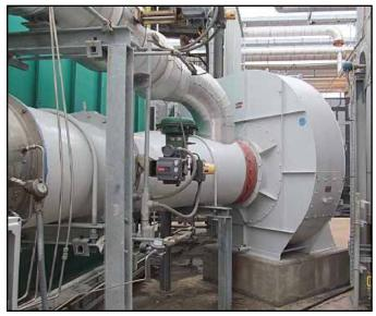
choice. A boiler blower air inlet operates under negative pressure, therefore the material chosen isn't strong enough for this application. Although this material is lower in price than other materials, it collapses under vacuum and punctures easily because it is very thin. The tear caused cold air to leak into the boiler blower, and dramatically reduced the efficiency of the boiler costing the operator money.
