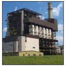
filter system.) To accommodate the dust hopper below, ESPs are typically 10 to 25 feet above the ground. The optimal temperature of the steam gas ranges from 280°F to 320°F. This particular ESP was operated in the only lignite or brown coal power station in Louisiana. It produces 650 megawatts of electricity.
