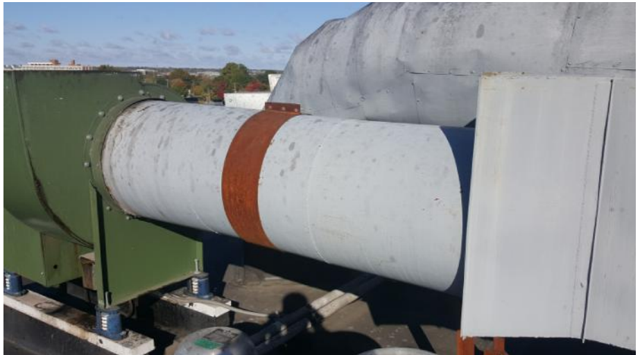
The ductwork before the expansion joint was installed
